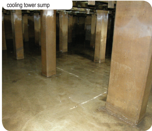
cooling tower sump
